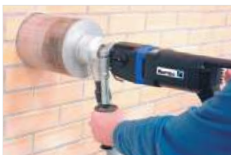
Messa in opera
